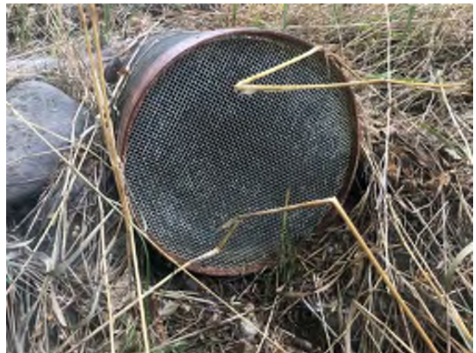
Photo 10 – Drain/Overflow outlet for Springs 3 – 5. No signs of sand, gravel, or hard water deposits.
