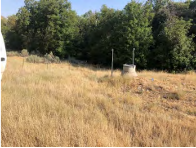
Photo 1 - Spring 2 Collection Box, looking northwesterly down the canyon, perpendicular to groundwater flow.
