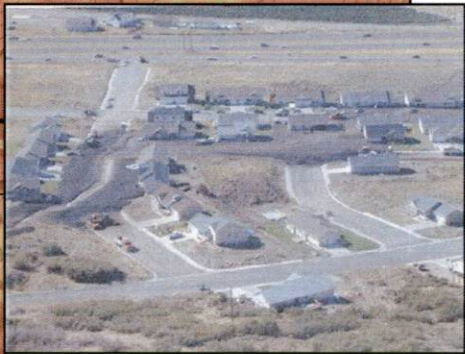
2002 Mud Slides Impact on Santaquin Homes
