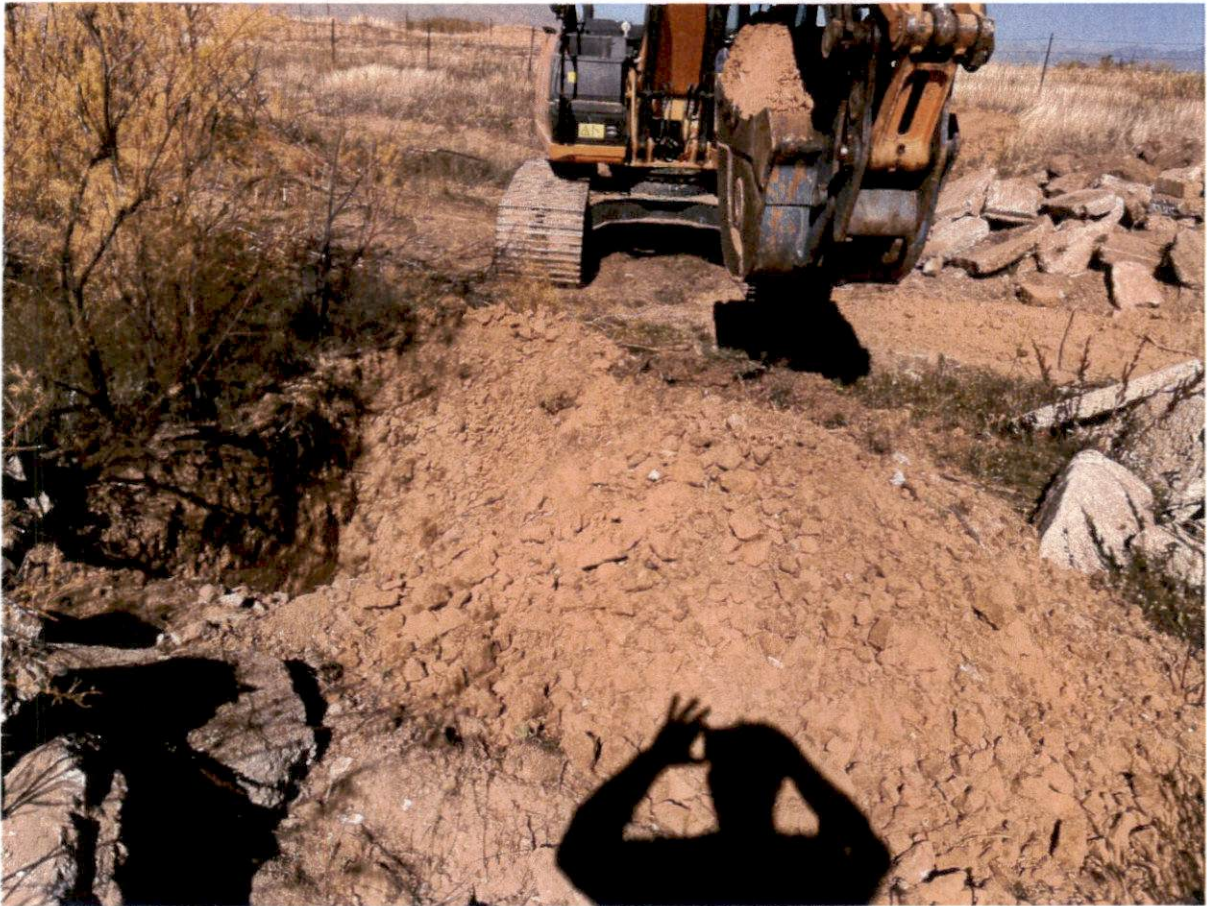
Hole 5 looking northwest. Tighter silt.
