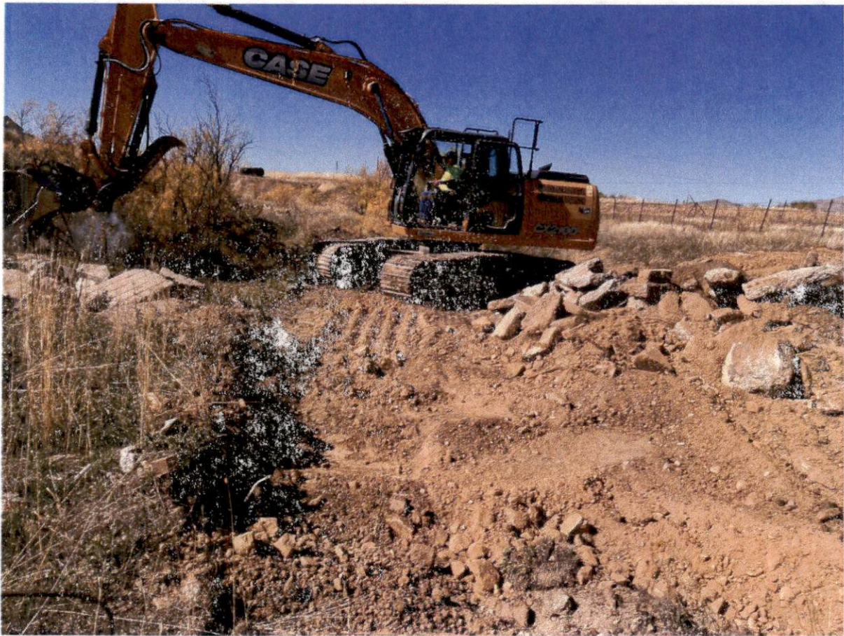
Looking west-northwest at the start of Hole 5. Trench between Holes 2 and 3 that are backfilled is shown.
