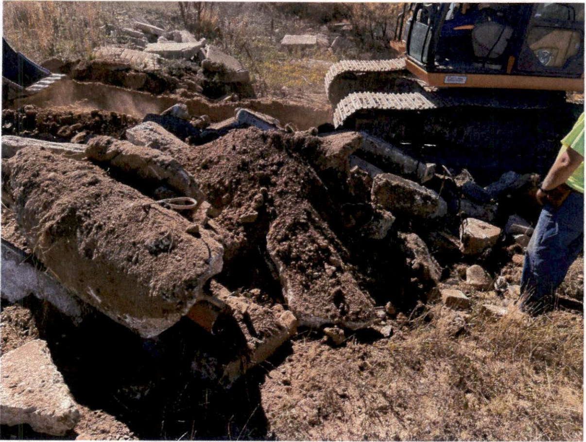
Looking south at trench between Hole 3 and Hole 4. Surface concrete and rebar pile scraped to side to dig down 10 feet and verify that there is not something buried below the surface piles.
