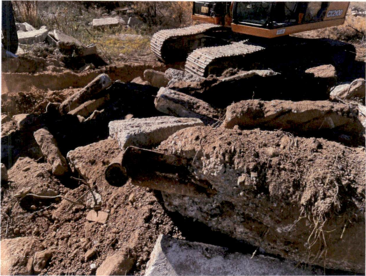
Looking south at trench between Hole 3 and 4. Note some rebar and metal gate post embedded. All material scraped at surface.
