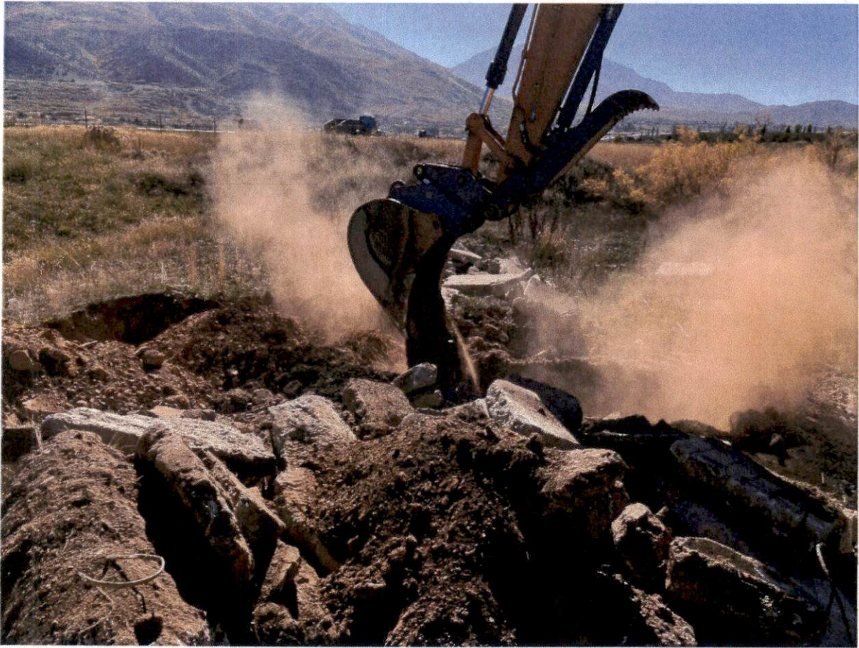
Filling trench between Holes 3 and 4. All surface debris left on surface for construction contractor to remove.
