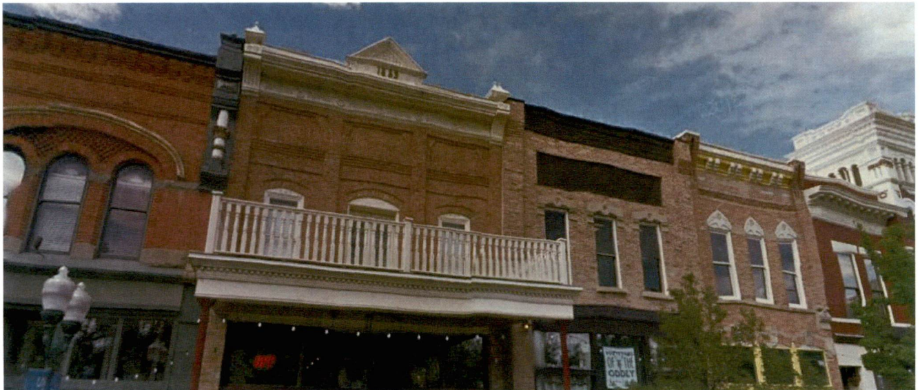
Figure 24. Parapets in Provo, UT.
